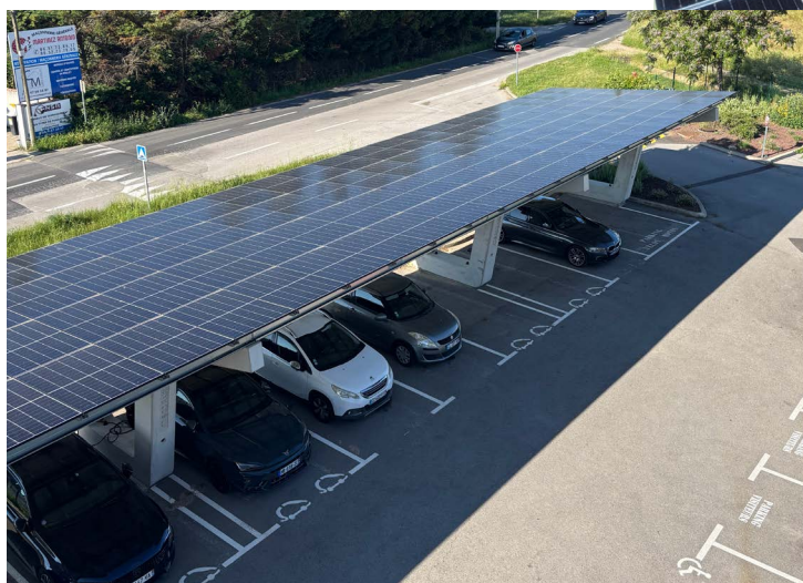
Commissioning in August 2025
